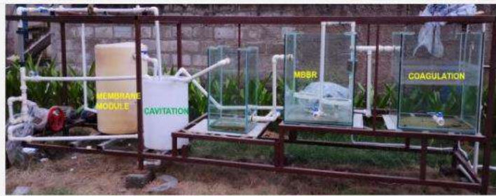
Figure 2 Pilot-scale setup installed at Prime Textiles, Rampur
